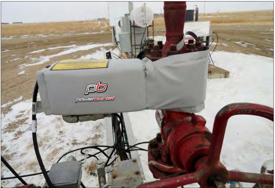
On-site Valve & Instrumentation Heater
