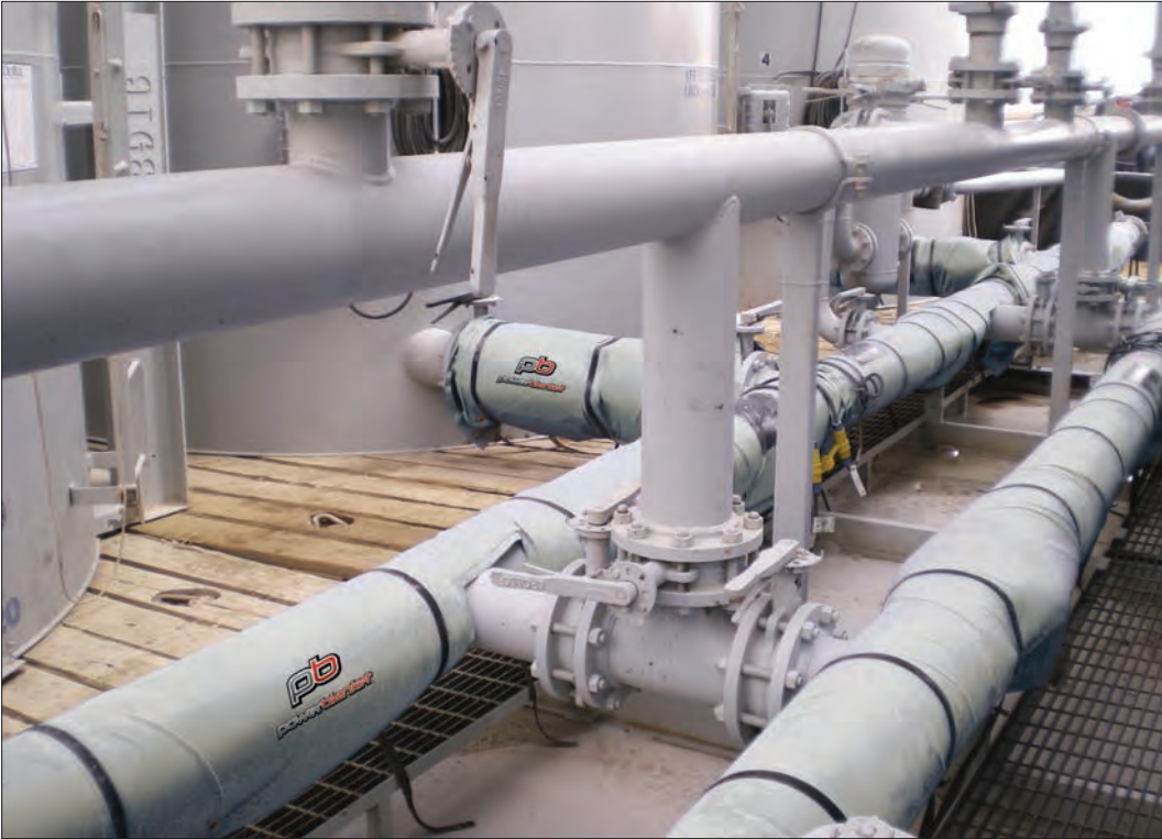
On-site Pipe & Manifold Heating System
